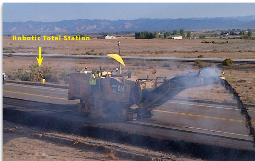
The antenna extending above the umbrella canopy on the milling machine receives wireless communication from the robotic total station. The operator controls the lateral movement of the machine, but the vertical movement is guided by AMG. The track height adjusts automatically to meet the profile, milling to an elevation 6 inches below the finished grade.
