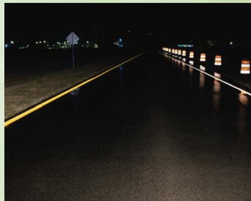
All-Weather Pavement Markings
