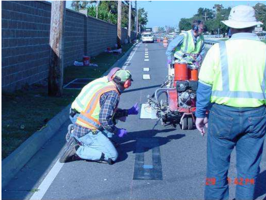
Figure 3. Illustration of test line installation procedure at Right Wheel track location.
