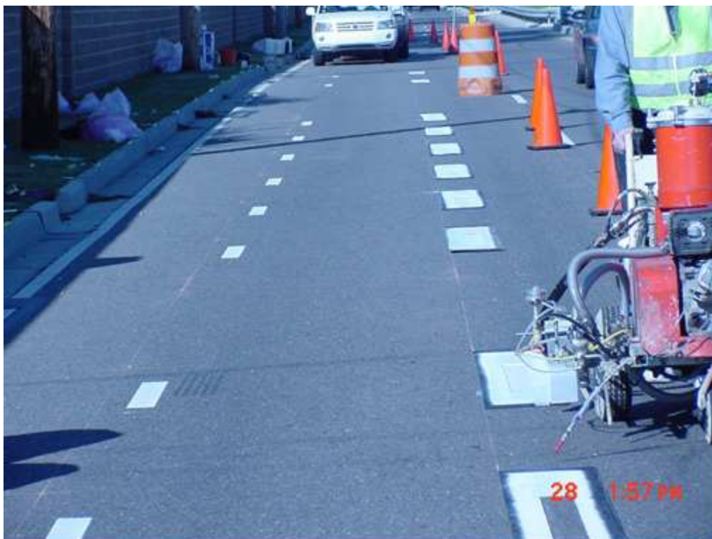
Figure 4. Illustration of paint line application showing masks used for 4' x 3' test lines
