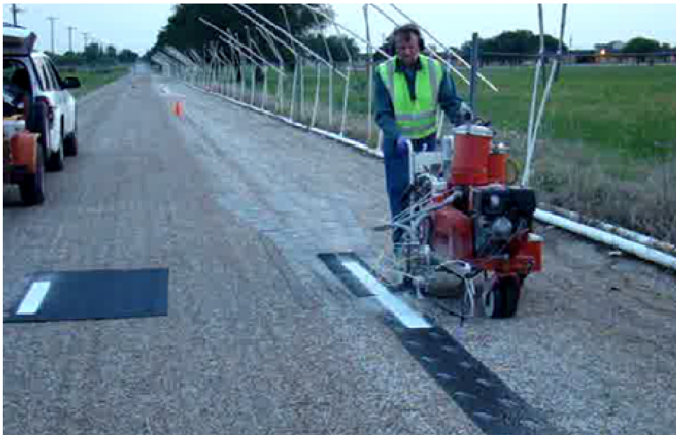
Figure 9. EZ Liner walk behind application cart used to apply painted lines
