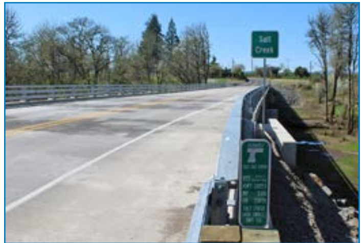
The Salt Creek Bridge was one of several internally cured bridge deck projects the Oregon DOT surveyed that showed significantly less shrinkage cracking versus traditionally cured concrete decks.
